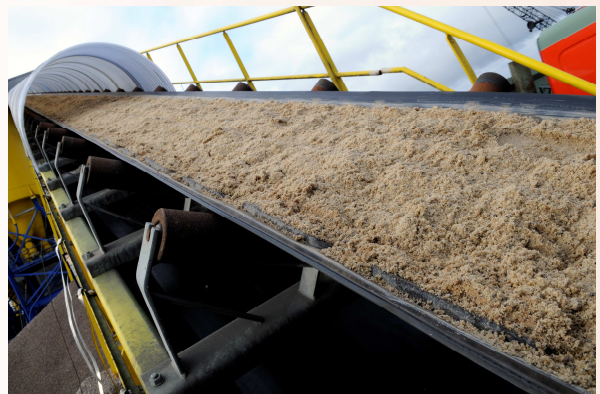
Misaligned drums and idlers cause extra wear
